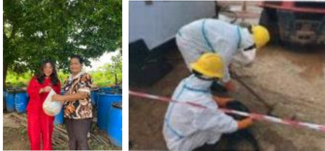
▲Working site of the Thailand project
