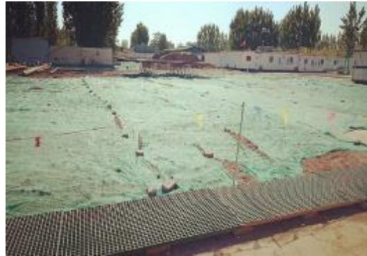
▲ Laying dust-proof nets at construction sites
