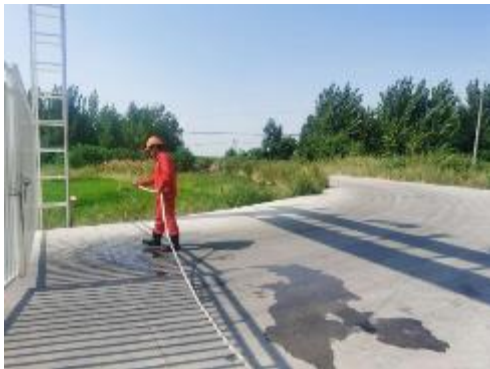
▲ Spraying water at well sites to reduce dust
